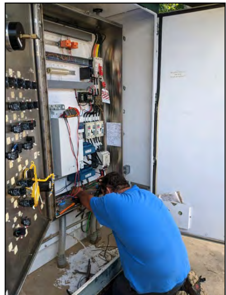
Staff continually works on facilities to keep everything operational. Here a mechanic rewires a faulty control panel.
