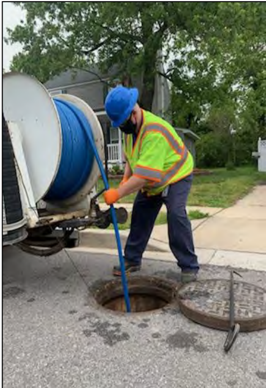
Clearing and cleaning sanitary sewer lines is ongoing, even in the midst of a pandemic.
